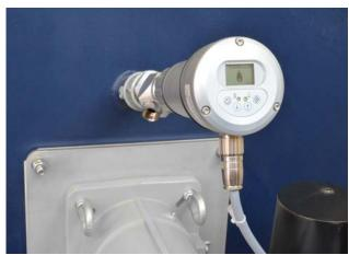
The LAMTEC F300K flame scanner in operation.
